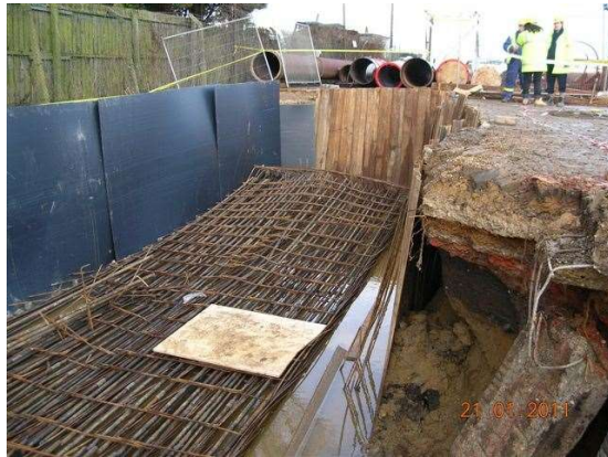
After the collapse
