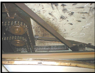
Asbestos panelling cladding escalator handrail drive adjuster
