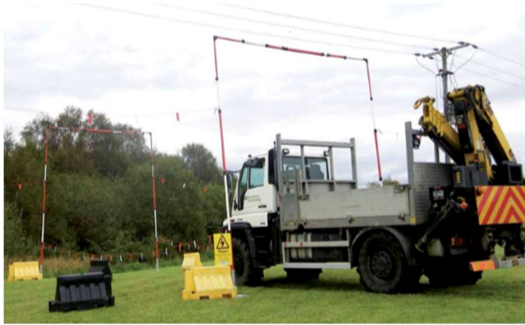
Figure 5 Typical passageway through barriers
