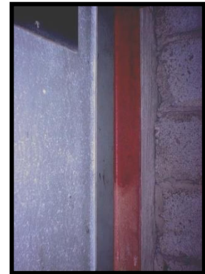
Asbestos panelling on the back of landing doors
