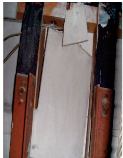
Asbestos as cladding within lift machine rooms
