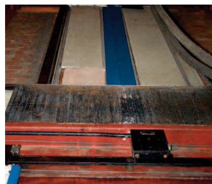
Asbestos on lift door panelling
