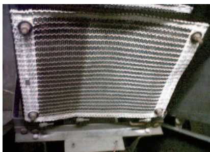
Resistor bank - rear of panel
