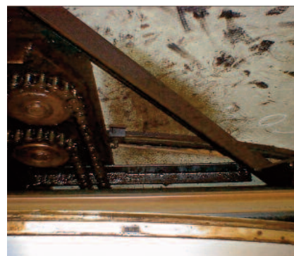
Asbestos panel within an escalator
