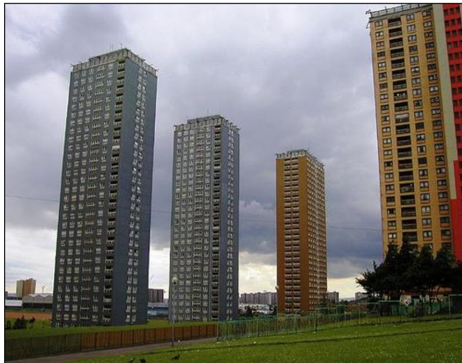
Example residential tower - Source: http://ukhousing.wikia.com/wiki/Tower_block
